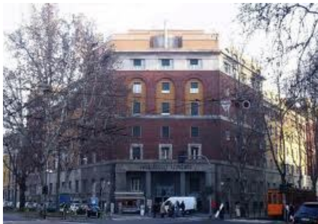
Figure 51: The Leonardo da Vinci Residence in Milan, Italy
