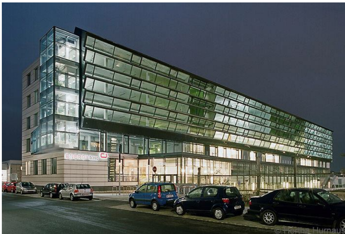
Figure 31: The ENERGYbase office building in Vienna (©Hertha Hurnaus)
